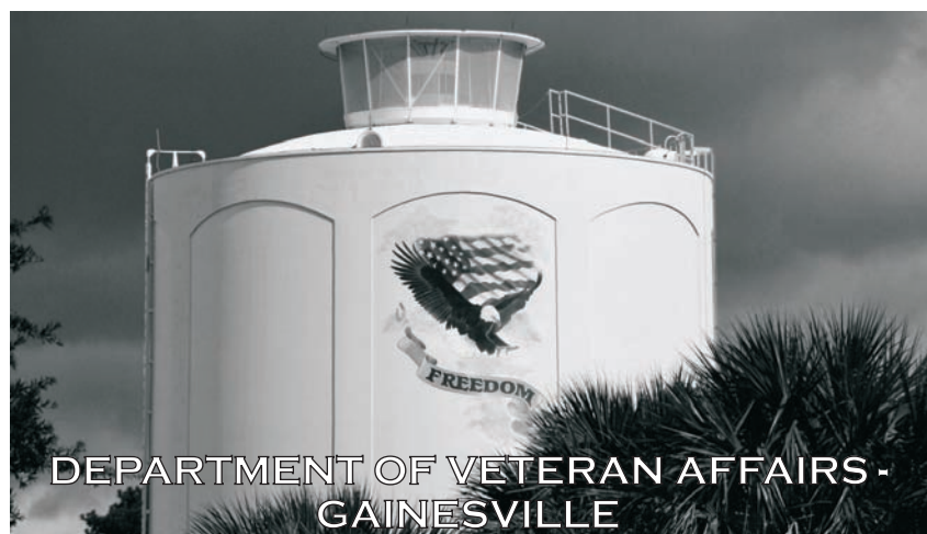
CITY OF PORT ST. LUCIE 2.0 MG WATER STORAGE TANK REISS ENGINEERING, INC.
