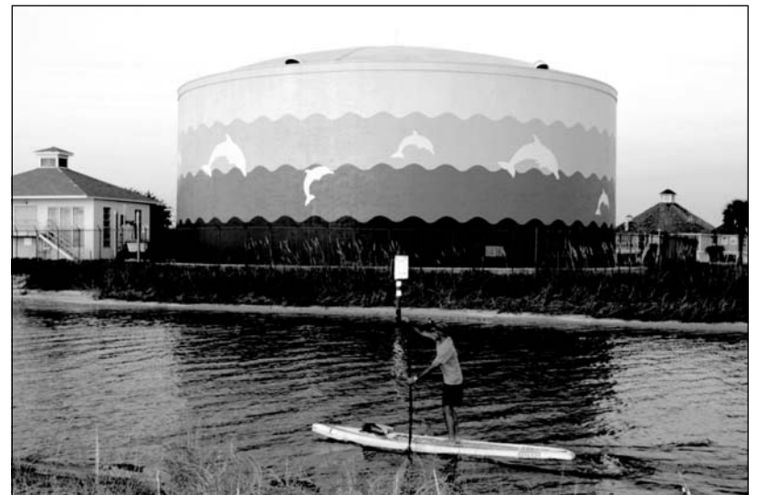
EMERALD COAST UTILITIES AUTHORITY - PENSACOLA BEACH, FLORIDA 3.0 MG POTABLE WATER STORAGE TANK CONSULTING ENGINEERS: BASKERVILLE-DONOVAN, INC.
