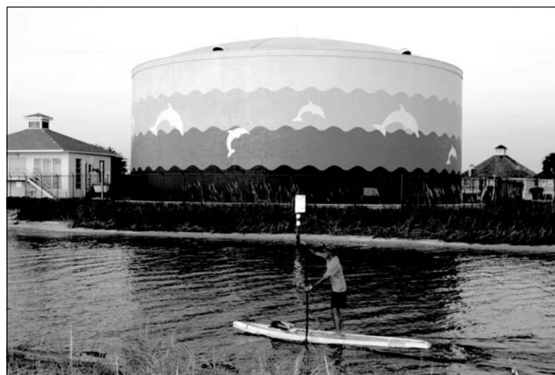
EMERALD COAST UTILITIES AUTHORITY - PENSACOLA BEACH, FLORIDA 3.0 MG POTABLE WATER STORAGE TANK CONSULTING ENGINEERS: BASKERVILLE-DONOVAN, INC.
