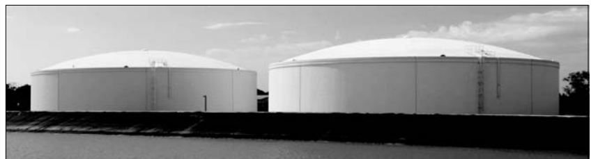
MANATEE COUNTY - SOUTHWEST WRF Two - 10.0 MG RECLAIMED WATER STORAGE TANKS CONSULTING ENGINEERS: AECOM
