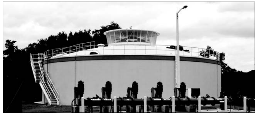
POLK COUNTY - IMPERIAL LAKES WTP 1.0 MG POTABLE WATER STORAGE TANK WITH 3800 GPM AERATOR CONSULTING ENGINEERS: JONES EDMUNDS AND ASSOCIATES, INC.
