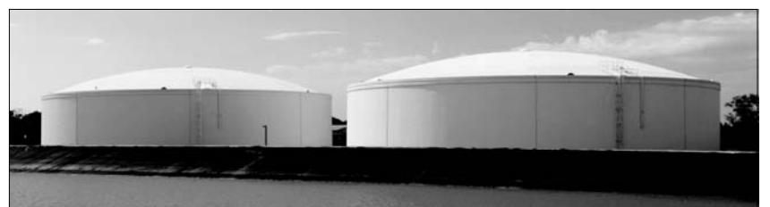
MANATEE COUNTY - SOUTHWEST WRF Two - 10.0 MG RECLAIMED WATER STORAGE TANKS CONSULTING ENGINEERS: AECOM
