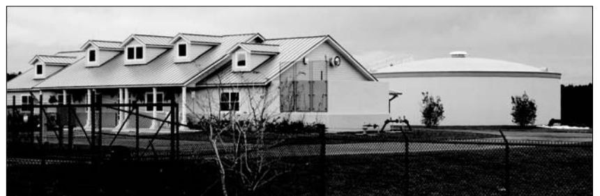
FLORAL CITY WATER ASSOCIATION 0.5 MG POTABLE WATER STORAGE TANK CONSULTING ENGINEERS: COASTAL ENGINEERING ASSOCIATES, INC.
