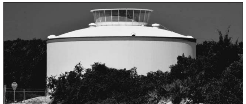
ST. GEORGE ISLAND WATER SYSTEM 0.6 MG POTABLE WATER STORAGE TANK WITH 2600 GPM AERATOR CONSULTING ENGINEERS: LES THOMAS CONSULTING ENGINEERS
