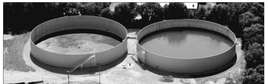
EMERALD COAST UTILITIES AUTHORITY TWO 5.0 MG STORMWATER COLLECTION TANKS CONSULTING ENGINEERS: WARRINGTON; JEHL-HALSTEAD, INC.
