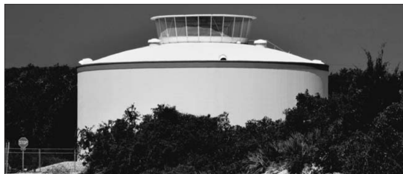
ST. GEORGE ISLAND WATER SYSTEM 0.6 MG POTABLE WATER STORAGE TANK WITH 2600 GPM AERATOR CONSULTING ENGINEERS: LES THOMAS CONSULTING ENGINEERS
