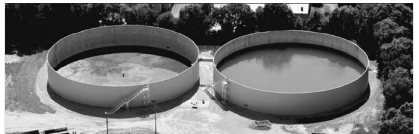
EMERALD COAST UTILITIES AUTHORITY TWO 5.0 MG STORMWATER COLLECTION TANKS CONSULTING ENGINEERS: WARRINGTON; JEHLE-HALSTEAD, INC.
