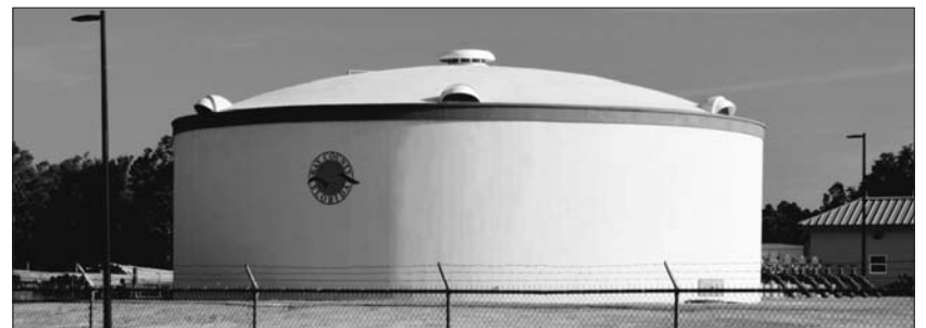
BAY COUNTY - SOUTHPORT 0.5 MG WATER STORAGE TANK CONSULTING ENGINEERS: PANHANDLE ENGINEERING, INC.
