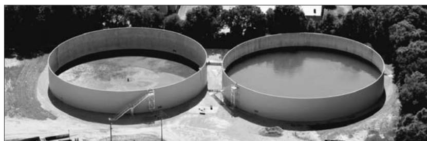
EMERALD COAST UTILITIES AUTHORITY TWO 5.0 MG STORMWATER COLLECTION TANKS CONSULTING ENGINEERS: WARRINGTON; JEHL-HALSTEAD, INC.
