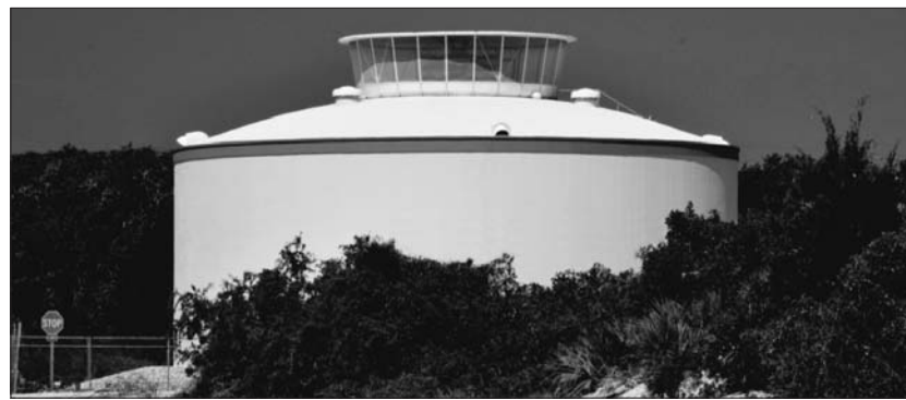
ST. GEORGE ISLAND WATER SYSTEM 0.6 MG POTABLE WATER STORAGE TANK WITH 2600 GPM AERATOR CONSULTING ENGINEERS: LES THOMAS CONSULTING ENGINEERS
