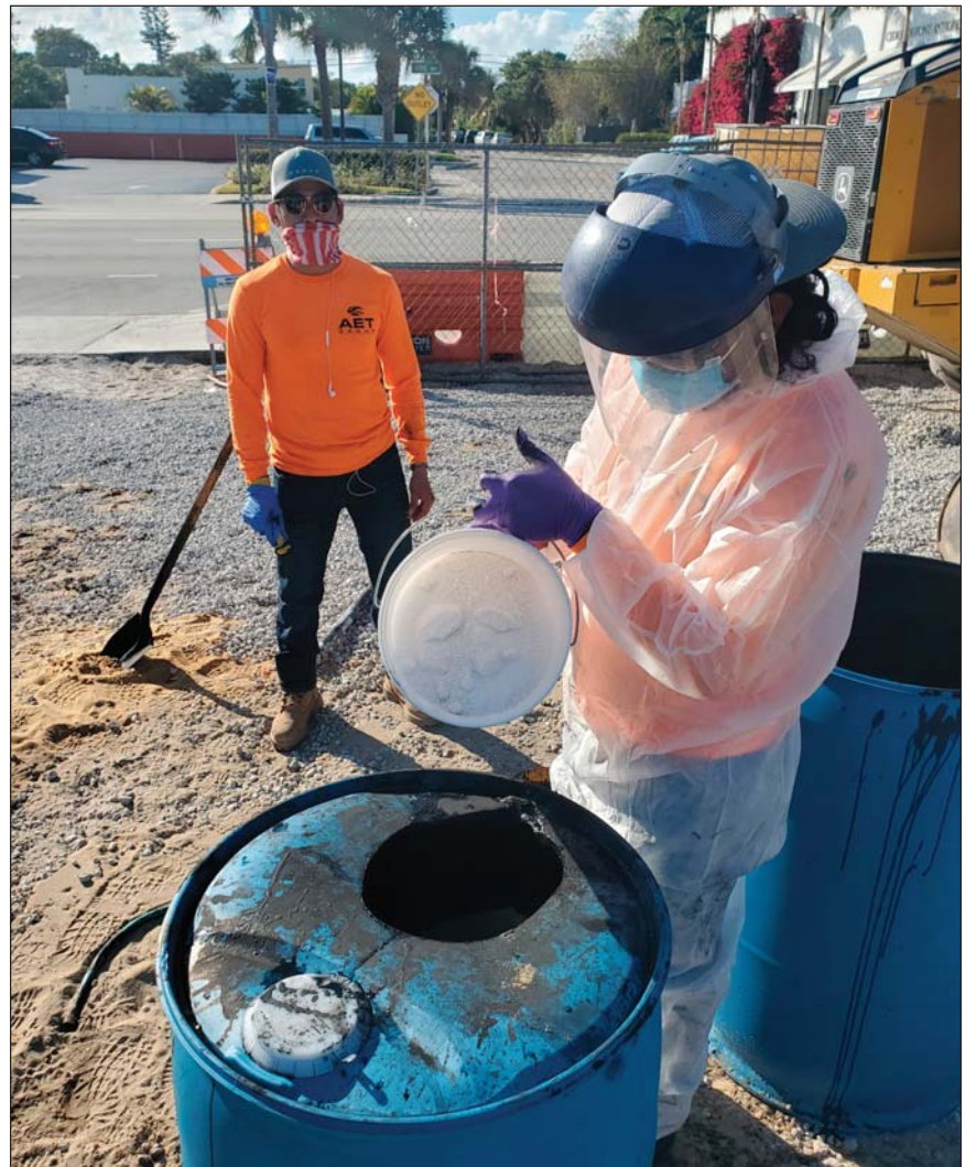
Photo courtesy of Advanced Environmental Technologies LLC
