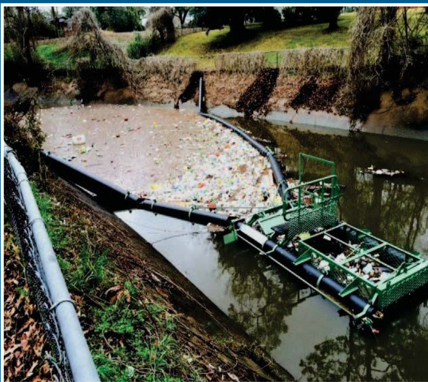
Bandalong Litter Trap™ In-Stream Trash Trap
